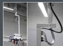
Special suspension with integrated power cord ensures vertical installation of E-BOX.
